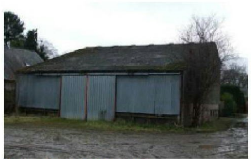
Above - Former barn materials
